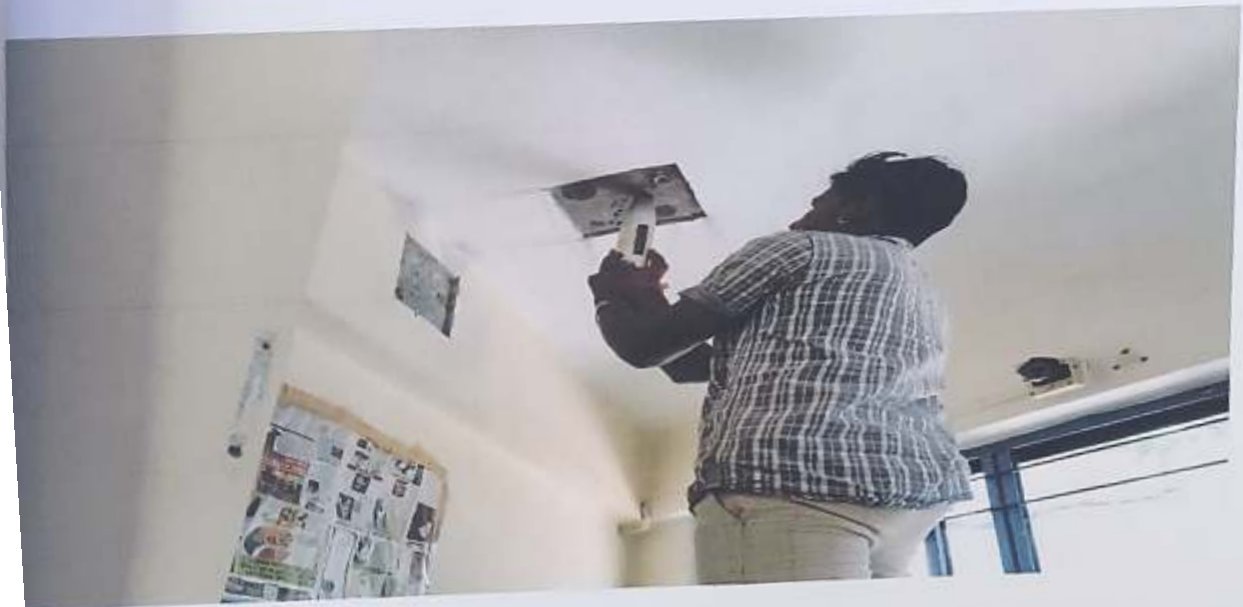
Rebound Hammer test
